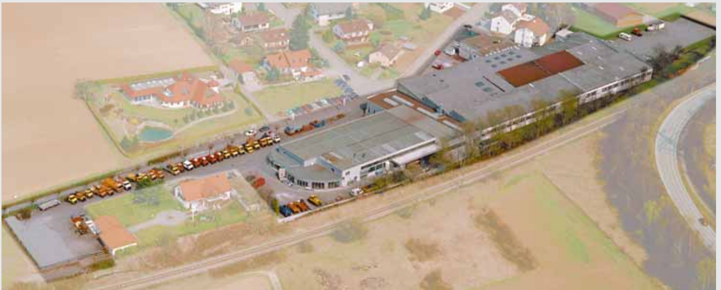
Air photo: ZAGRO production facilities and administration building
