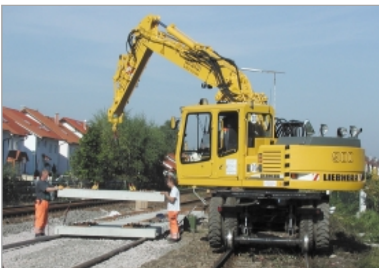
Liebherr excavator working with crane on railway tracks.
